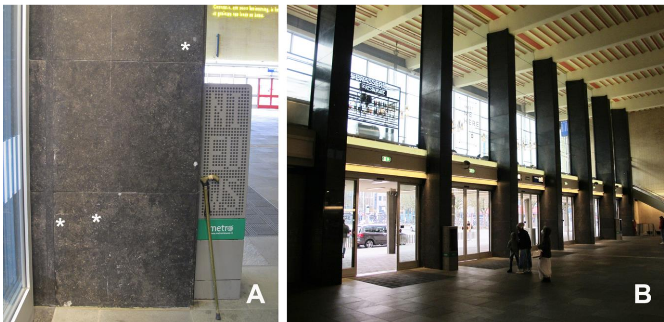
Fig. 1. Mississippian limestones of Eindhoven station, the Netherlands. A , The facing stones that include the specimens discussed herein, marked by (*). Upper right = Fig. 2A; lower left = Fig. 2B; centre left = Fig. 2C. The cane is about 92 cm long. B , General view of the main exit to the station; the pillar on the right side of the nearest (far left) exit contains the crinoids discussed herein.
